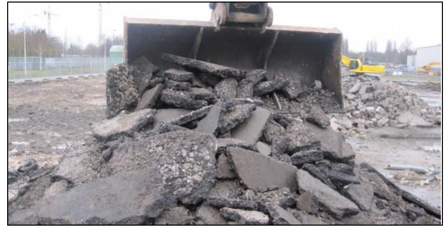
Asphalt with high % recycled materials
