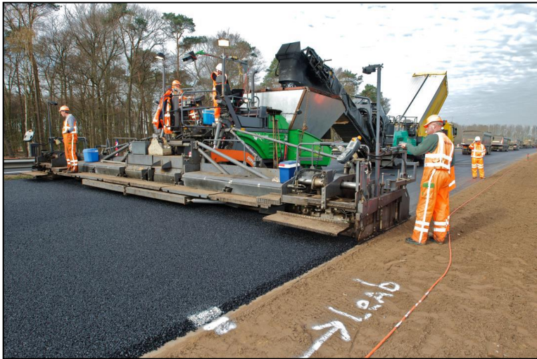
Low Energy Asphalt
